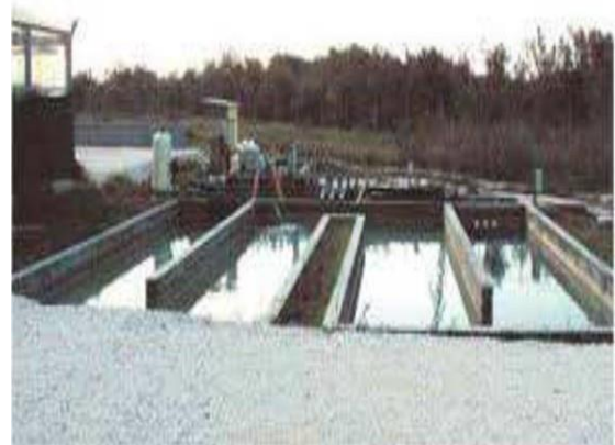
Figure 5b: Rectangular Sedimentation tank (Al-kizwini, 2015)
