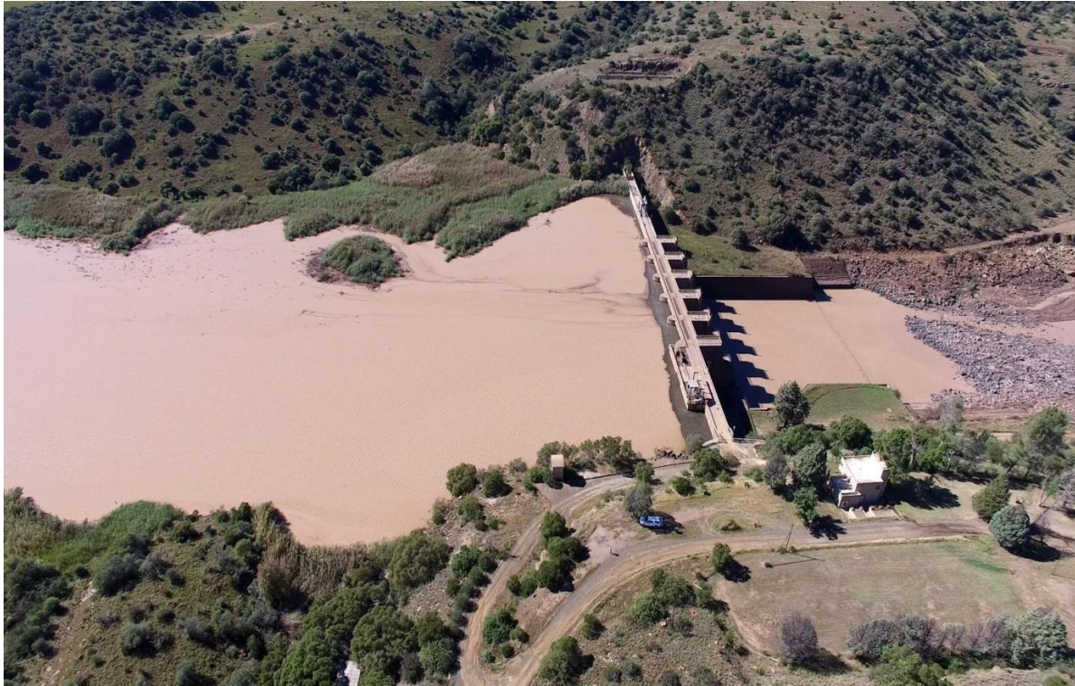
Figure 4: View of Welbedacht Dam with so much silt (Sancold, 2018)
