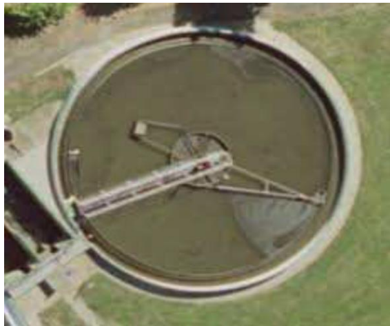
Figure 5a: Circular Clarifier (Al-kizwini, 2015)
