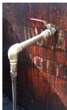
Figure 9: Tap fit to the tank for O&G removal
