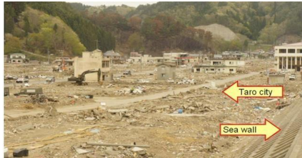
Figure 10. The Devastation Caused by the 2011 Tsunami Source: Kiuchi (2019)
