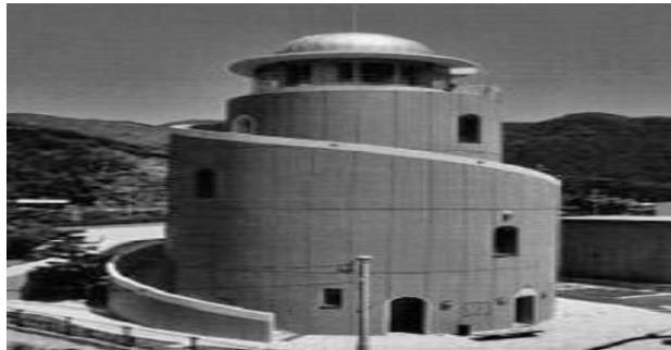
Figure 9. Escape Building in Japan
