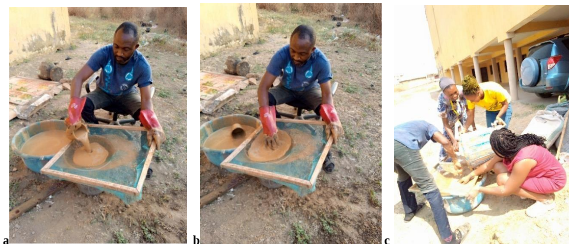
Fig. 3(a); (b) & (c). Process of sieving clay
